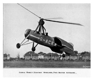
The power or thrust of autogyro comes from a powered propeller (or in later designs a jet engine) meaning that most do require some take off runway, but normally only tens of feet. As they can land in an equally small space, the autogyro had distinct advantages over airplanes as they are much more manoeuvrable and stable flying at low speeds, but can also fly faster than the helicopters. The autogyro is unable to "stall" in mid-air, making it considerably safer than other aircrafts.
